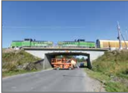
FIGURE 5.1.1 A RAILWAY CONCRETE TROUGH BRIDGE IN HAPARANDA, SWEDEN, WAS STRENGTHENED BY POST-TENSIONING OF BARS PLACED IN HOLES DRILLED TRANSVERSELY THROUGH THE BRIDGE SLAB. THE ALLOWABLE AXLE LOAD COULD BE INCREASED FROM 250 TO 300 kN. © MAINLINE CONSORTIUM
