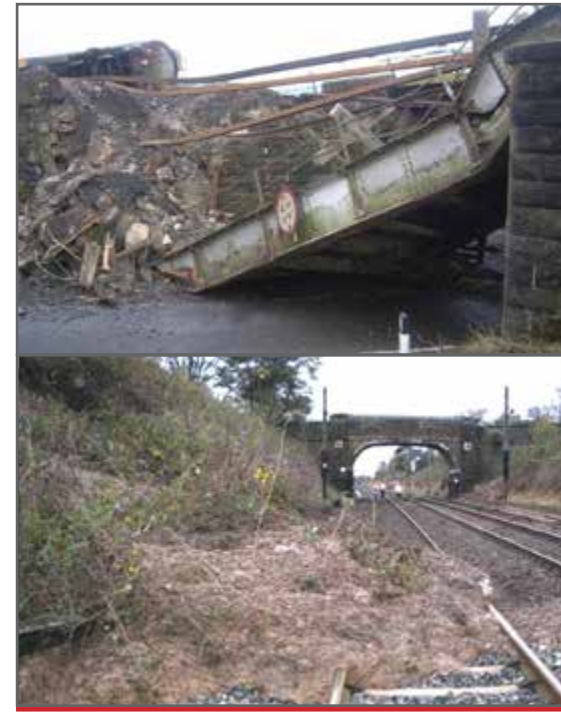
FIGURE 2.1 COLLAPSE OF STEWARTON BRIDGE IN SCOTLAND AND EARTHWORK CUTTING FAILURE. © MAINLINE CONSORTIUM
