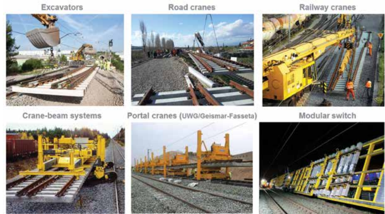
FIGURE 6.3 DIFFERENT TECHNIQUES FOR TRACK RENEWAL. ©MAINLINE CONSORTIUM
